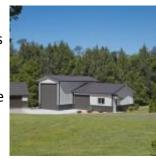
One creative aspect that our customer requested was 3' perimeter wainscoting around the entire building with HardiePlank® lap siding. Other accessories that were added per our customer were 18" eave and gable overhangs, 10' continuous flow ridge vents, one for each building and a PermaBilt® awning with enclosed soffit over his man door.
